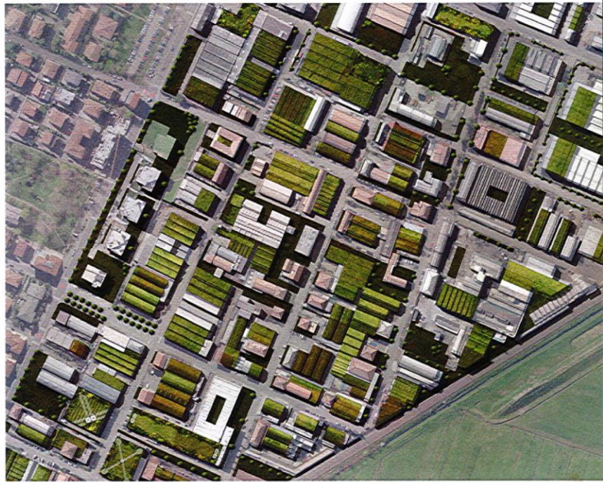
1. Simulation environment and application of the index of the productive area of the Villaggio Artigiano - central area
